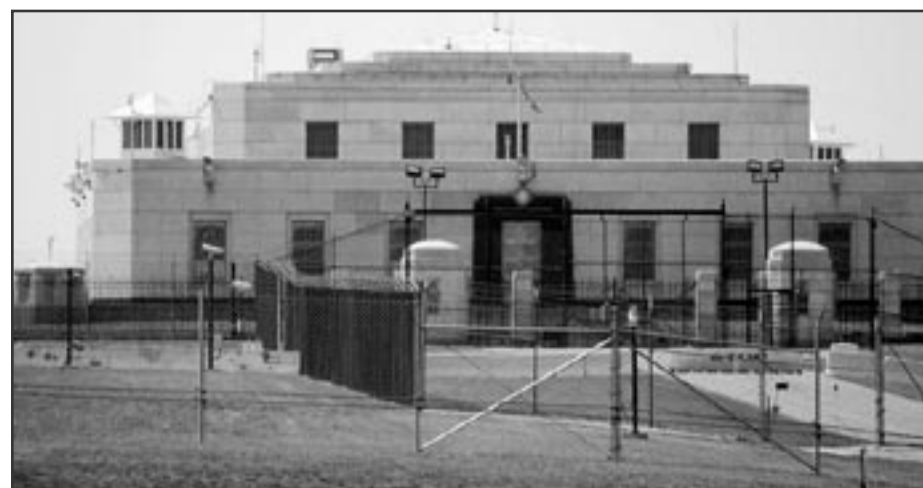
Fort Knox Gold Depository
